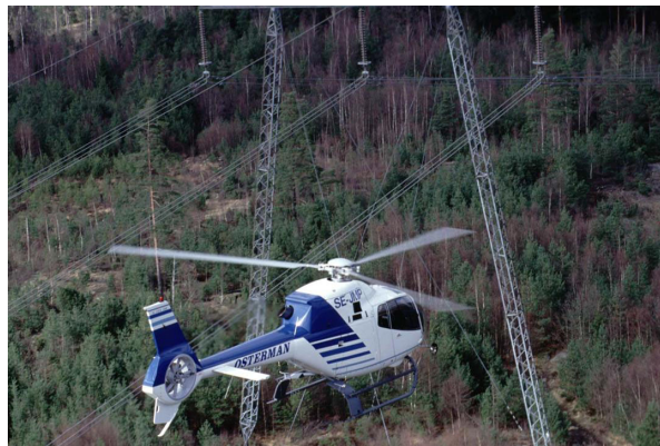
Power line inspection
